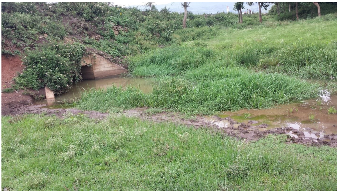
Figure 39 Bridge Over the Awuside River
